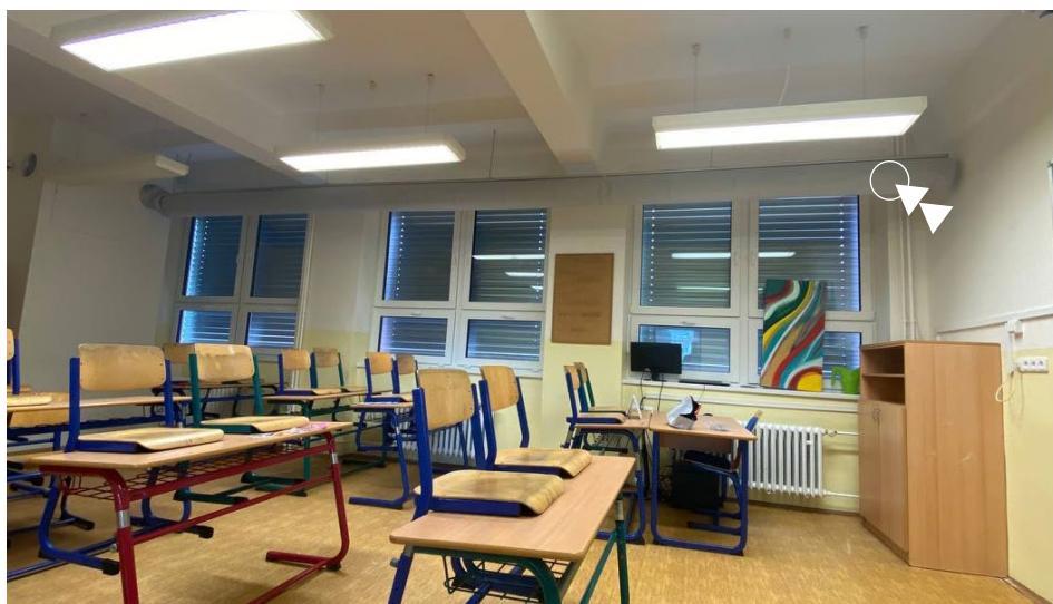
Local unit in the classroom with fabric diffusers - controlled supply of fresh air
