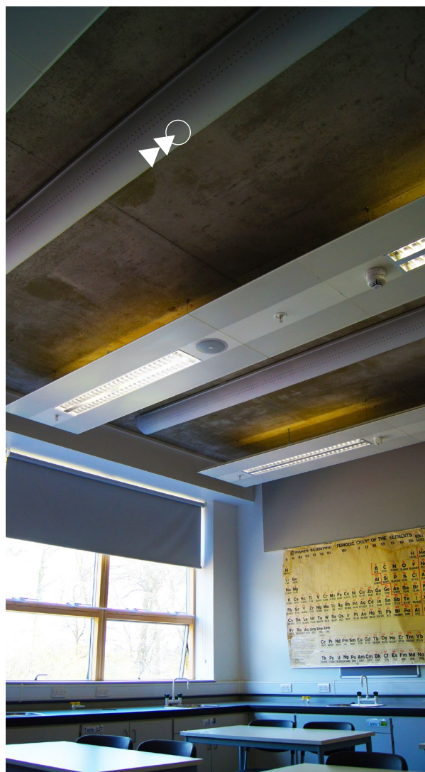
Local unit in the classroom with fabric diffusers - controlled supply of fresh air
