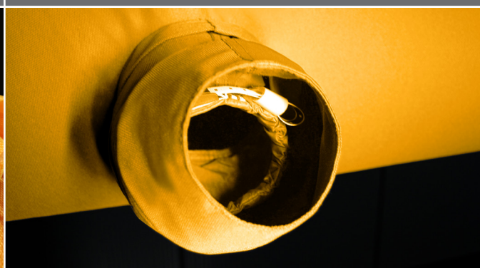
Damper for air volume correcting
