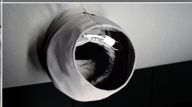
Damper for air volume correcting
