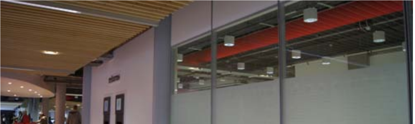
Smaller system ventilates a sorting and administration area
