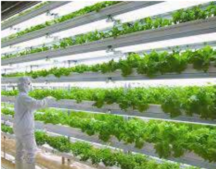
Vertical diffuser systems with precision, rack-level air distribution for top-to-bottom temperature and humidity consistency in any size vertical grow operation
