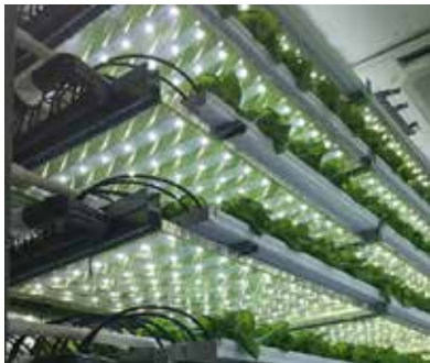
Vertical diffuser systems with precision, rack-level air distribution for top-to-bottom temperature and humidity consistency in any size vertical grow operation
